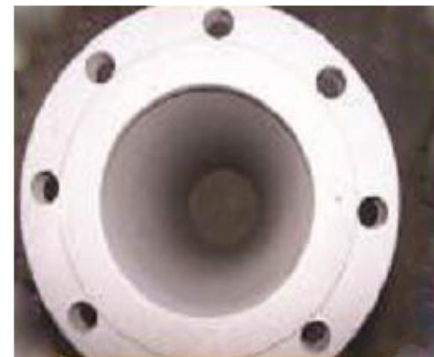
Chemically Cleaned Line
